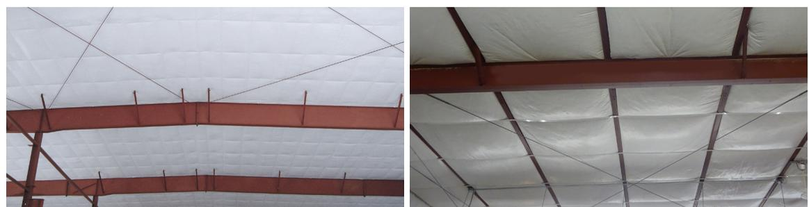
Liner system roof assembly (left) shows single piece vapor retarder encapsulating purlins versus long tab assembly (right) shows each vapor retarder sealed atop framing, leaving purlins exposed.
